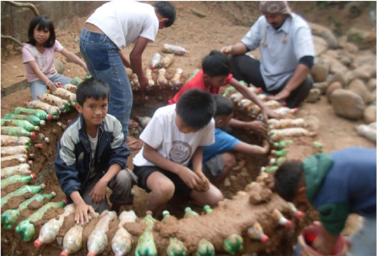
Illustration 11: Cob construction of the circle garden in the Balili Food Forest Playpark.
