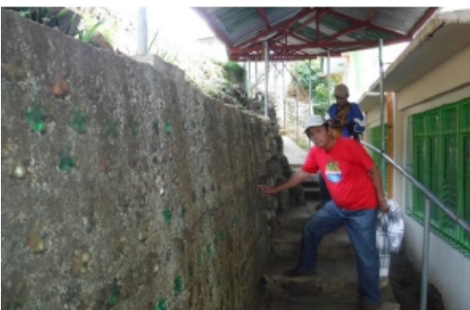
Illustration 16: Ecobrickens 'sunken' fully into wall and also protected from the sun by a roof. Great!
