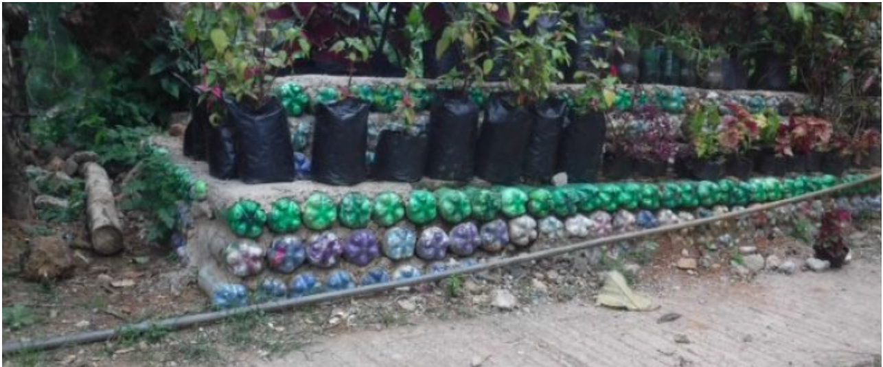
Illustration 8: Ecobricks were being used extensively around the school for garden borders. The school has developed a technique to minimize the use of cement to build with the ecobricks. No cob is used. However, the bottoms of the bottle have full sun exposure. Wear and degradation can already be observed. Ecobricks will be destroyed in only a few years.
