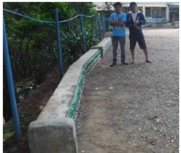
Illustration 9: The school was using ecobricks to make extensive school benches. This was one of the best techniques that we observed: a solid, nice looking bench. It might even be possible, given the thin mortar, to remove the ecobricks when this construction is destroyed. Still however, the bottoms of the ecobricks have excessive exposure to the sun.
