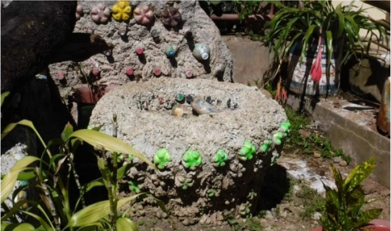
Illustration 22: A not so ideal use of ecobricks in Bali, Mt. Province. Caps show signs of fading and degradation. Ecobricks are fully stuck in cement and will not be able to be removed without being damaged.
