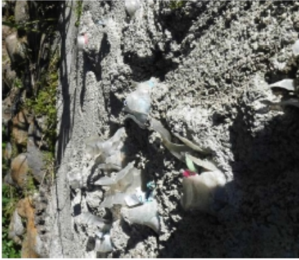
Illustration 12: Bottle tops exposed to sun have disintegrated. Bottle caps disintegrated first. Note cement cover up on ecobrick tops below.
