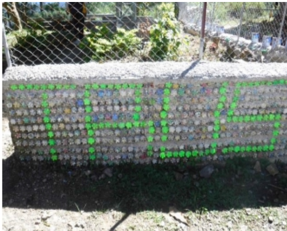
Illustration 18: Using painted ecobricks to make a pixelated ecobrick and cement sign
