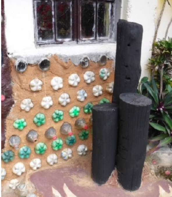
Illustration 3: Outdoor cob work (which is protected by an overhanging roof) continues to endure and look fantastic.
