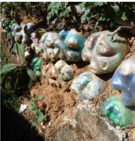
Illustration 15: In some places the cement render had fallen or most likely been broken away from the bench surface. In this case, some of the cob was beginning to erode and the exposed bottles, were beginning to fade and degrade.
