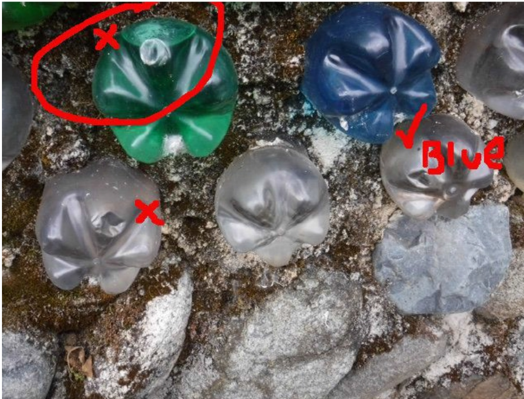
Illustration 7: Note the air bubble in the green bottle. Close inspection showed that the indent was degrading fast due to reflected sunlight. Note also the blue bottle-- this bottle contains no air bubble and has endured. The other grey bottles once contained color water. The water has either escaped or the color faded. Somehow the blue food coloring has endured unfaded for five years!
